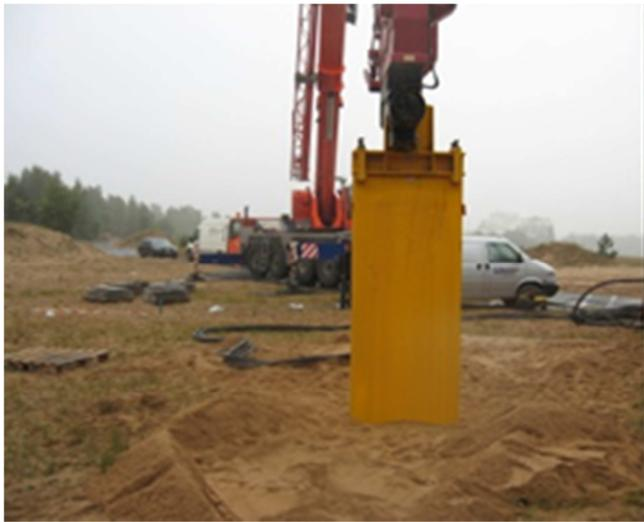
Fig. 6a Driving of installation box
